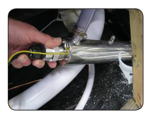
When replacement UV lamp has been installed, conduct a final leak check:
