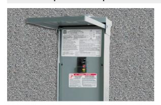
When the spa is filled to the correct level, turn on the power at the GFCI breaker. (Ensure that the 120V spas are connected to the proper electrical outlet.)
